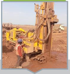
This technique is used when open voids that are present in rock mass with fluid matter. This reduces permeability by improving the shear strength, Also, this reduces deformability. It also helps to reduce the outward flow of water in high pressure water tunnels.
