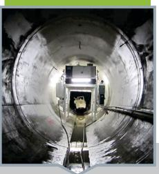
During the Tunnel Contact grouting process, grout is injected into voids between a tunnel liner and rock surrounding it. Additional consolidation of rock formation surrounding the tunnel is also achieved with this technique.
