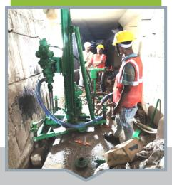
Curtain grouting is the technique where a curtain or barrier of grout is constructed to reduce permeability. It is done by drilling and grouting a series of holes.
