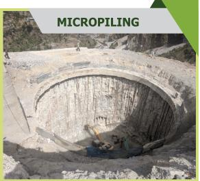
Micropiles are friction piles that run deep into the foundation. They are formed using strong steel casings. This piles helps in the load pressure to be transmitted to the soil around them.
